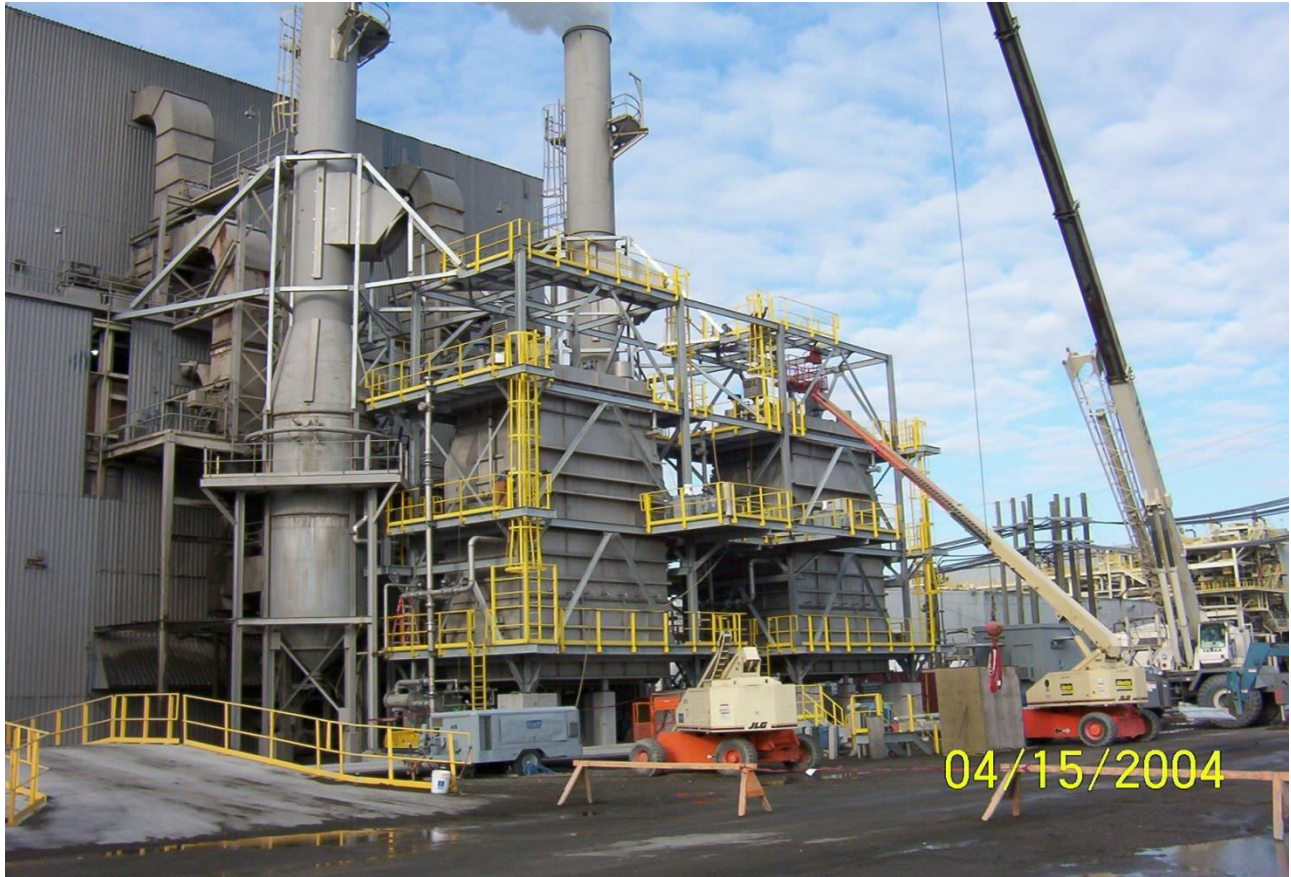
Figure 4-17 – Units 5&6 under construction
