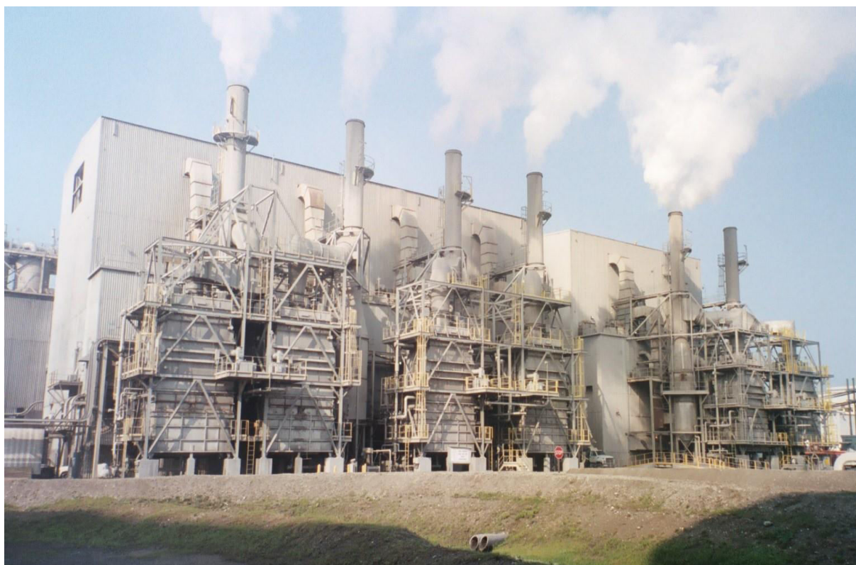
Figure 4-16 – WET ESP Array at PCS Phosphate
